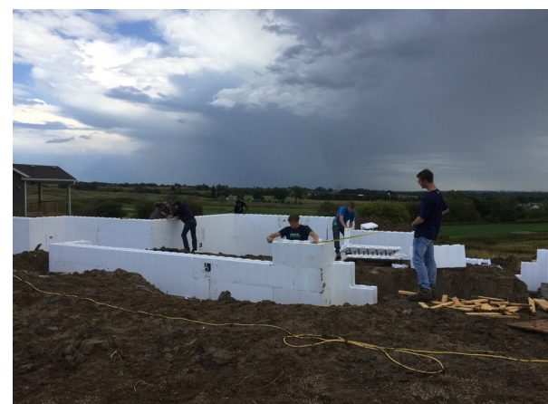
Vocational construction house work has begun
